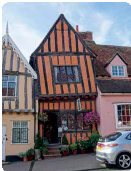
The crooked house at Lavenham.
