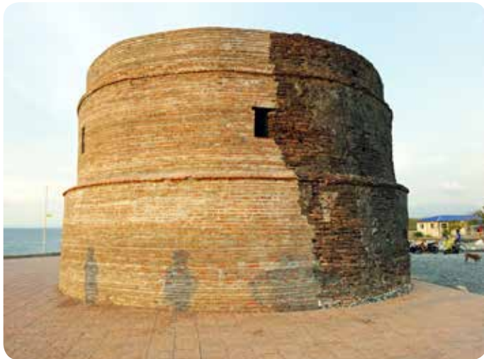
The Luna baluarte, showing its old (dark) and newly reconstructed (light) halves.
