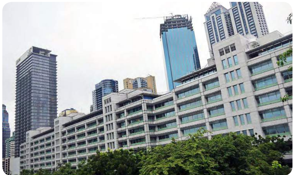
ADB's three atria, from the roof of the car park building. The new atrium is on the right.
