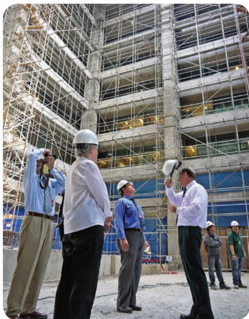
Inside the new atrium.
