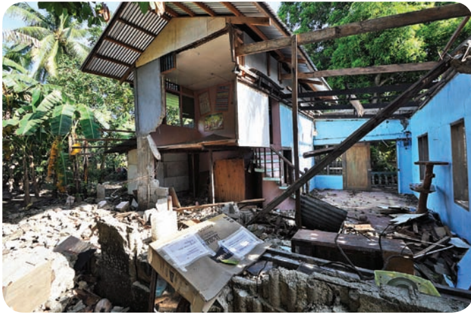
A village home destroyed by the quake
