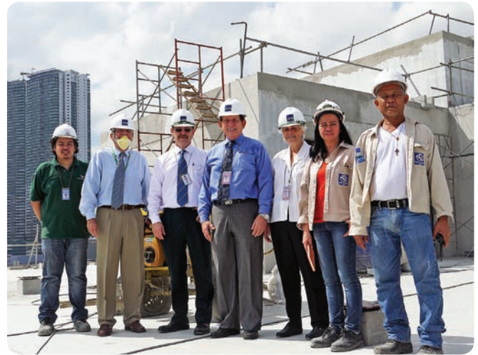
Touring the new atrium with the builders: l-r: Jerome Dañas (EEI architect), Hans-Juergen Springer, Anders C. Andersen (head of the project for ADB), David Parker, Jill Gale de Villa, Monette C. Cruz (EEI architect), and Felizardo Compacion (EEI engineer).
