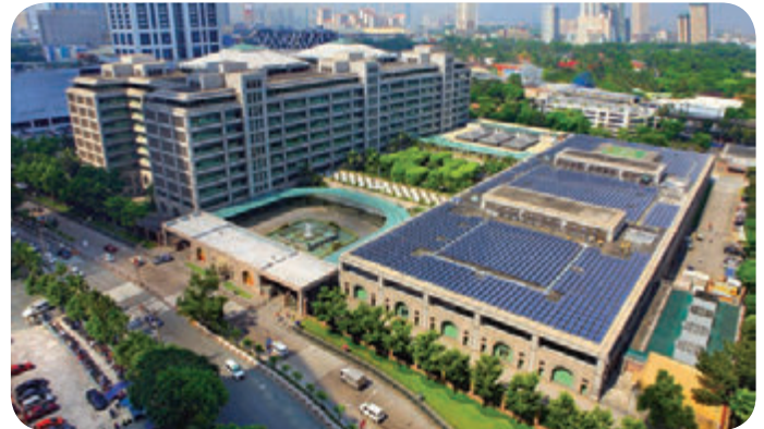
Solar panels on the roof of the Special Facilities Block.
