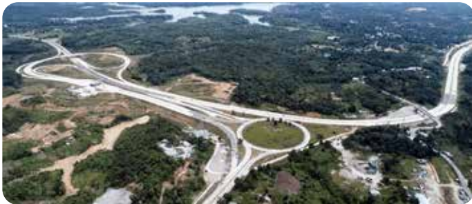
Completed toll road to Nusantara.
