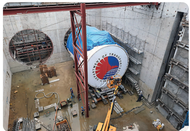
The Metro Manila Subway Project under construction.
