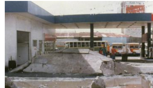
Rise of buried pipes, tanks
